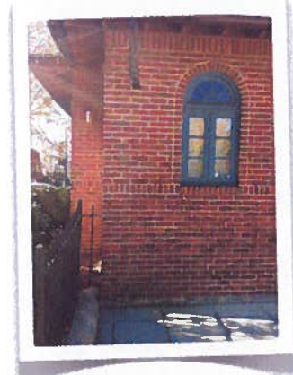
Downspouts missing
